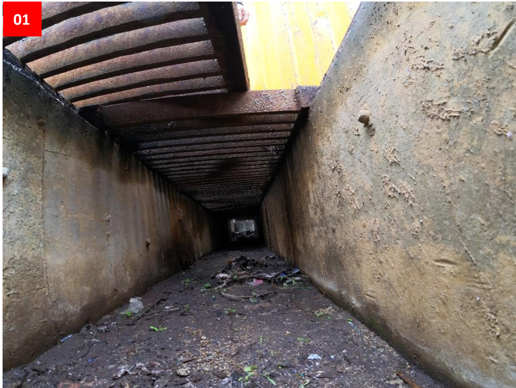
b) Site photo taken on 3.3.2026
